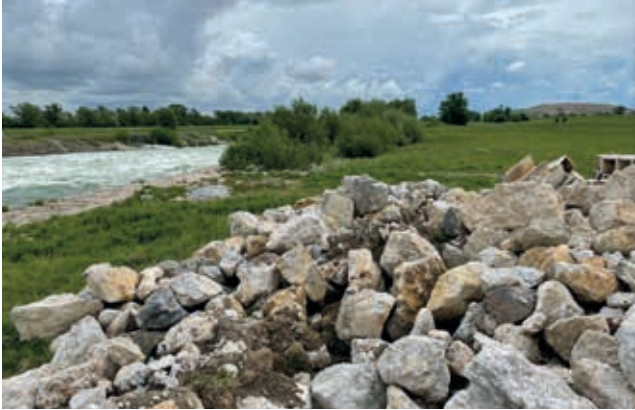
Figure 38: Rocks and stones prepared to secure the ramp.
