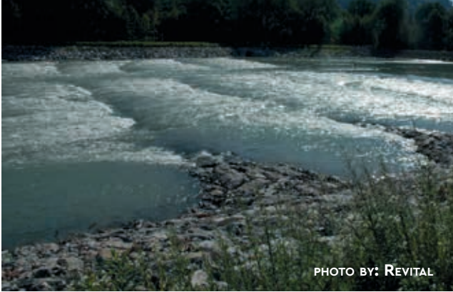
Figure 34: Flat fish passable ramp - best practice (Salzach at Freilassing, Austria/Germany).
